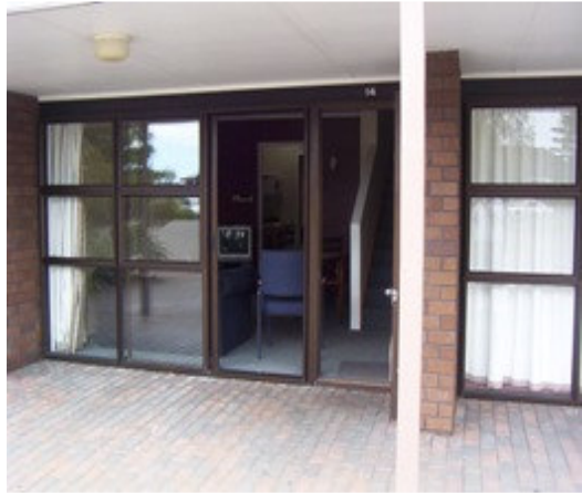
Unit entrance's, Enter direct to living area, With parking in front.
